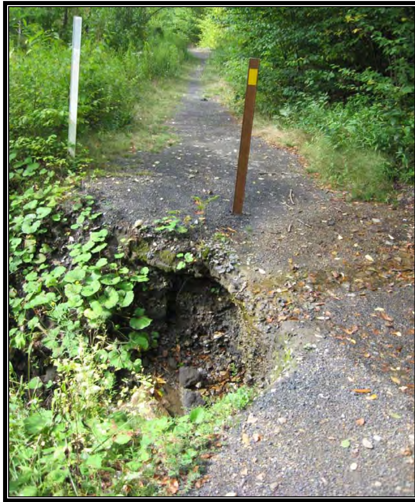
Figure 2. Example of erosion damage along the Blackwater Grade. AWP property is on the left, NFS land on the right. Conditions have already created a safety hazard and will continue to worsen without treatment.
