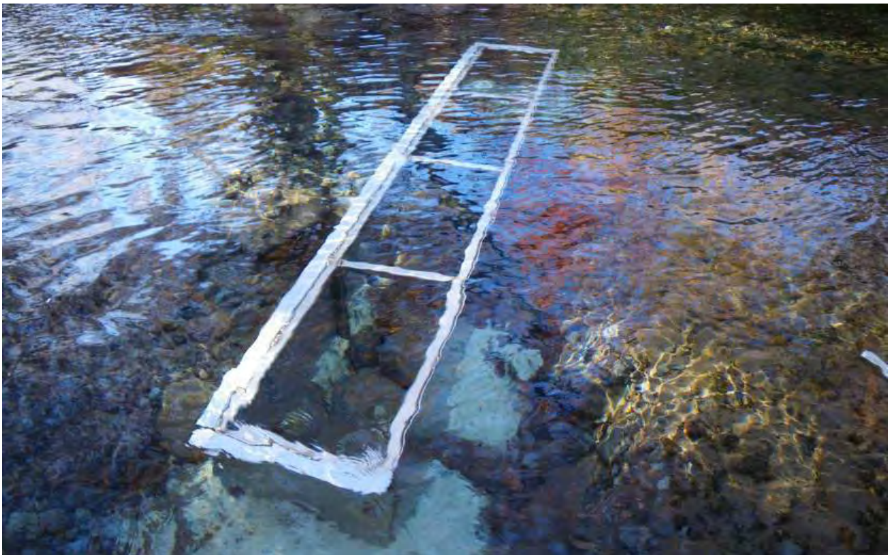
Figure 7 Construction of the velocity barrier portion of the crayfish barrier in Pond 5 of Sucker Springs Creek.
