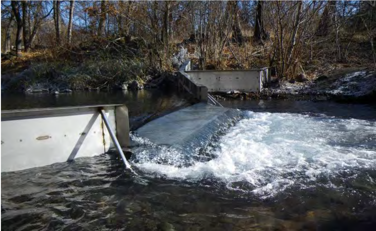
Figure 6 Operational crayfish barrier at Pond 4 of Sucker Springs Creek.
