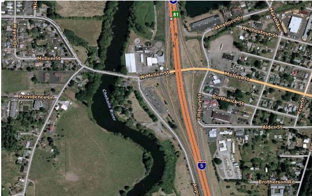
Figure A-1 Mellen Street Bridge
