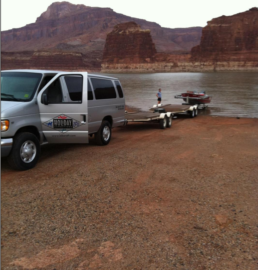
Hite Ramp, gravel extension, triple trailer coupling to launch hard hulled craft; Ramp slope approximately 2-3 degrees, solid substrate Tim Gaylord
