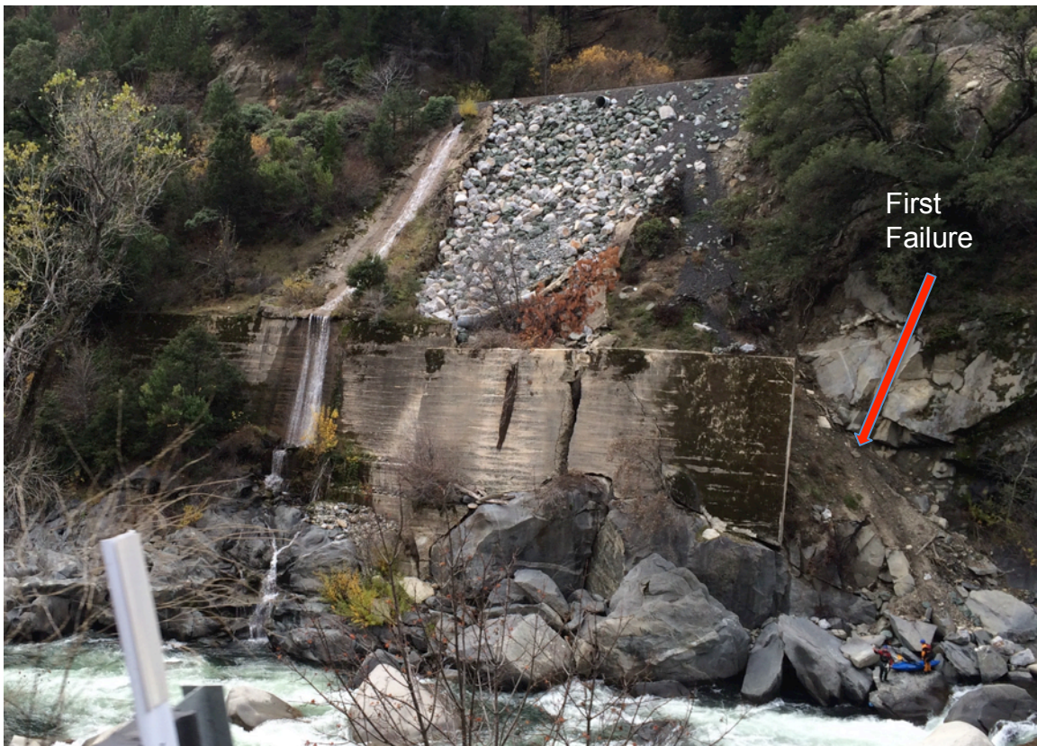
Image 2: December 5, 2016. View of first failure.
