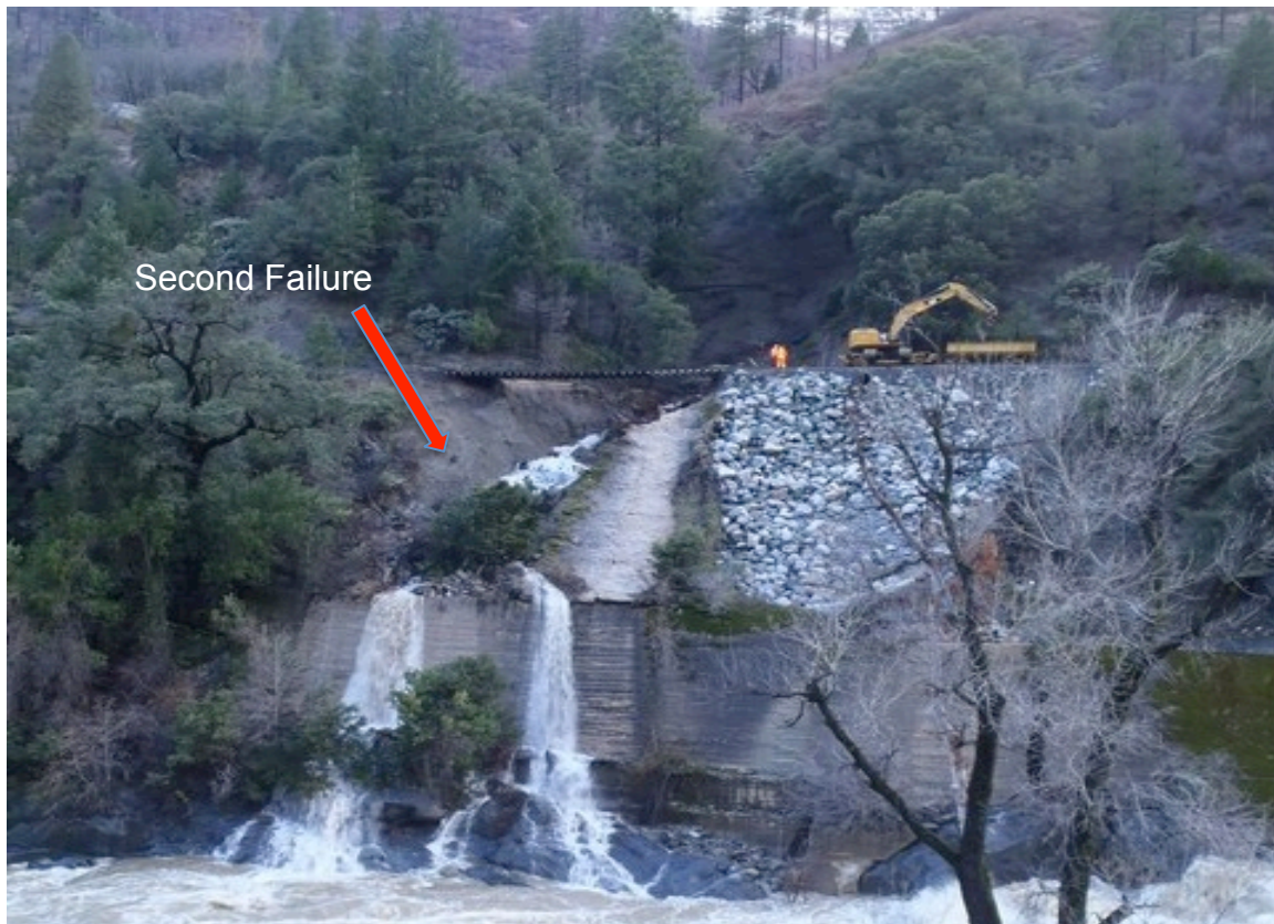
Image 4: January 12th 2017. Complete washout of the railbed.
