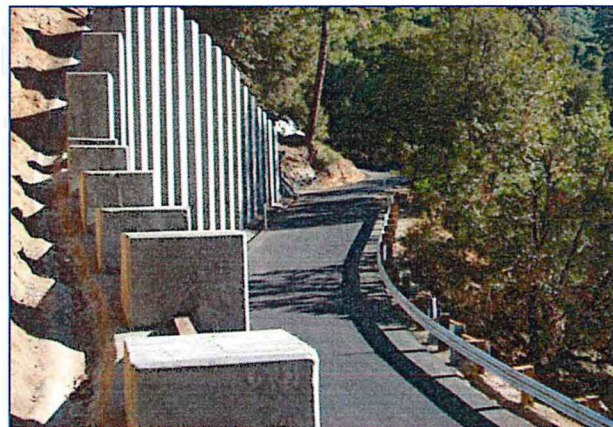
Soldier Pile Wall Constructed in 2007
