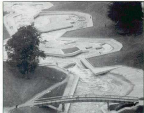
Figure 42. An "artificial river" near Nottingham, England which was first developed through physical modeling.
